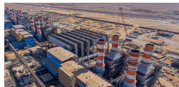
The Megaproject combined cycle plants, from the top: Beni Suef, Burullus, New Capital
