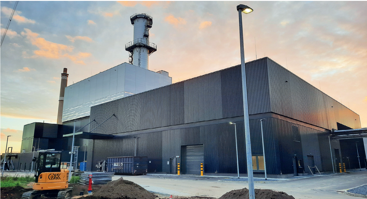
The new cogeneration plant from Vattenfall Wärme in Berlin-Marzahn proves that industrial facades do not have to be dreary: With the day's changing light, the CHP plant also changes its appearance
