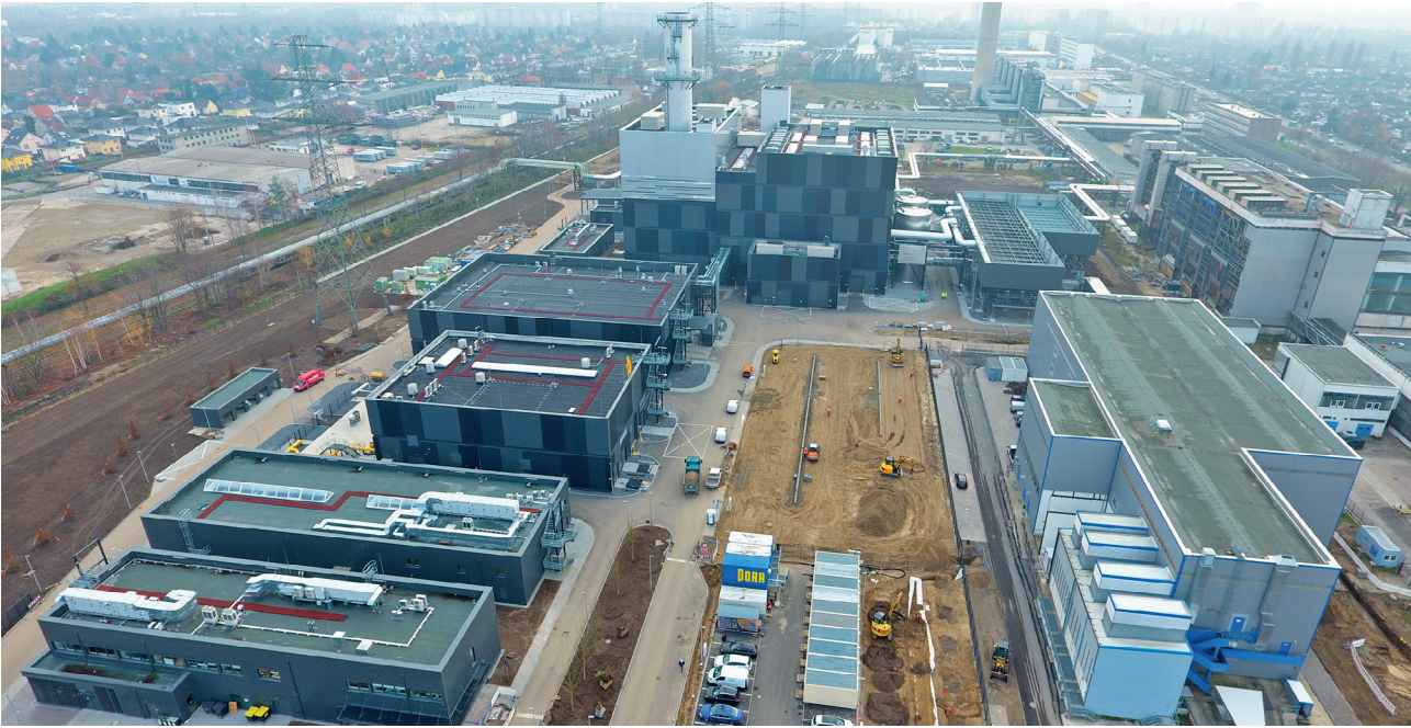
Figure 1. All tightly put together: The CHP Plant in Berlin-Marzahn was built on a small site due to clever planning and plenty of prefabrication
