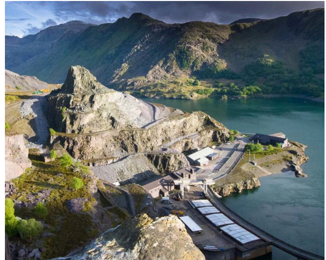
Dinorwig power station
