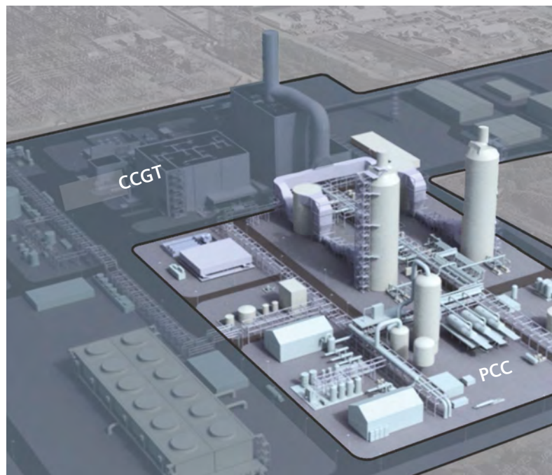
Figure 11: Typical installation of a PCC unit at a large CCGT power plant
