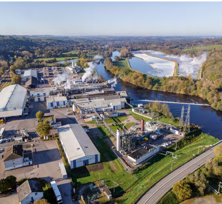
Figure 6: Cogeneration plant at Smurfit Kappa's paper mill, Saillat-sur-Vienne, where 100% H 2 operation was demonstrated
