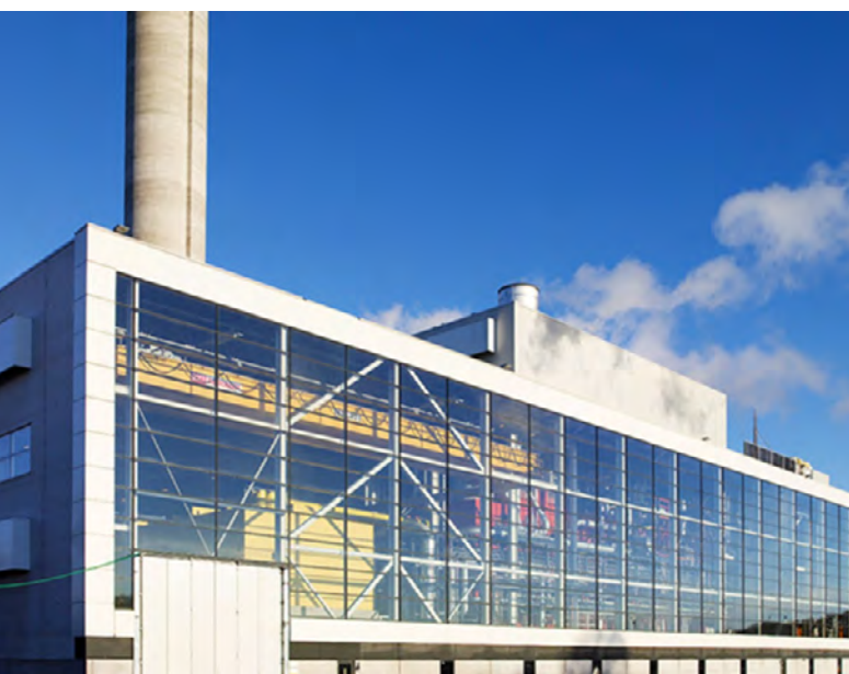
Figure 7: SGT-800 HVO100 demonstration at Göteborg Energi's Rya KVV (CHP) facility, 2021
