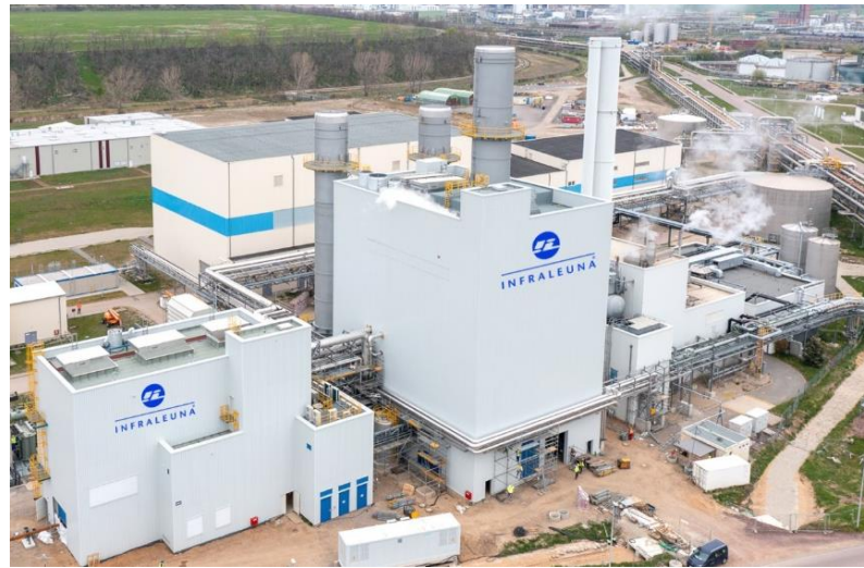
InfraLeuna's modern combined cycle power plant is located in Leuna, Germany.
