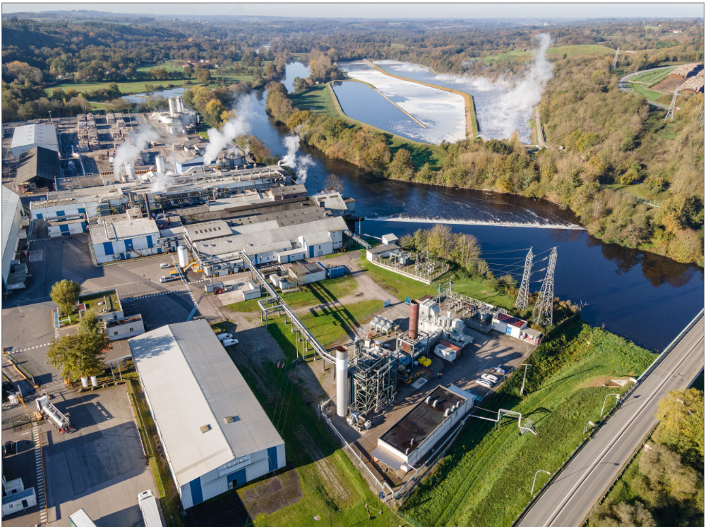
Figure 4. Smurfit-Kappa plant site. SGT-400 gas turbine driven CHP plant (center foreground) supplies 12MWe to the grid and 20MWth process heat to the plant. An electrolyzer, hydrogen compressor, and storage tanks were added for the HyFlexPower project.
