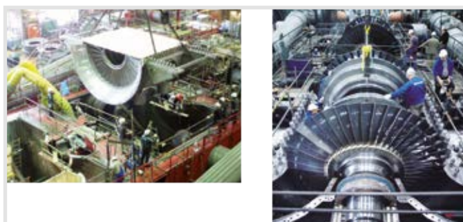
Fig. 6. Installation of modernized LP turbines.
