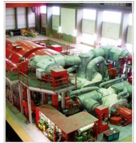
Fig. 8. Successfully modernized turbine generator set.
