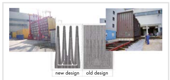
Fig. 7. Condenser module exchange.
