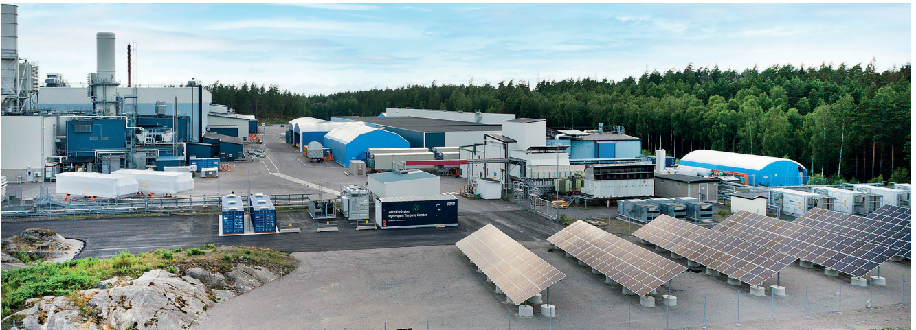
Above: View of the Siemens Energy plant in Finspång, location of ZEHTC. In the foreground is the photovoltaic system and behind that the electrolyser, with hydrogen tank, and the control room for battery storage
