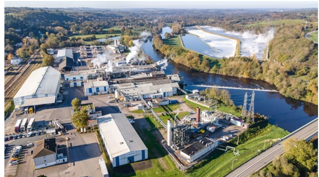
Figure 22: Smurfit Westrock SGT-400 Cogeneration plant in Saillat-sur-Vienne, France.
