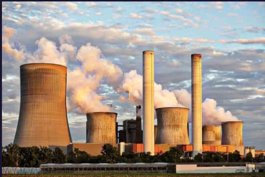
Conventional Coal Power Plant
