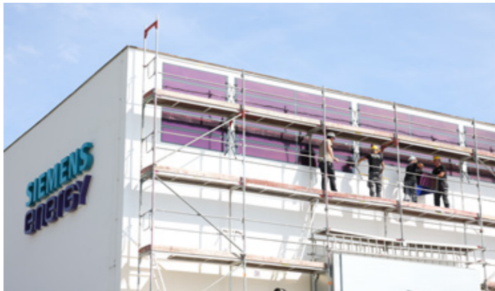
Installation of flexible photovoltaic film modules on Nuremberg power transformer factory.
