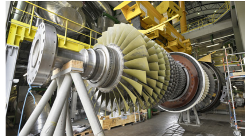
Gas turbine maintenance at the Donaustadt power plant.
