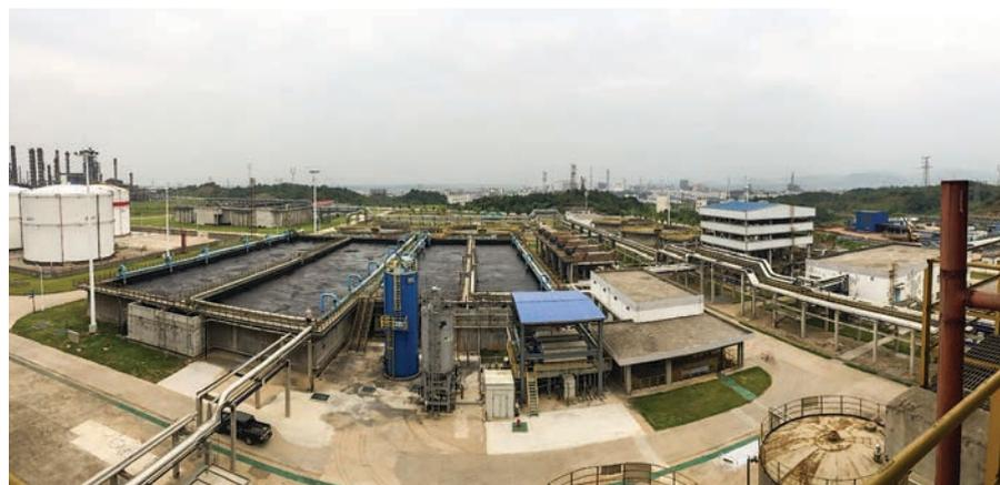
**FIG. 1.** The refinery's wastewater treatment process units include PACT biological treatment systems and a wet air regeneration (WAR) hydrothermal treatment unit.
