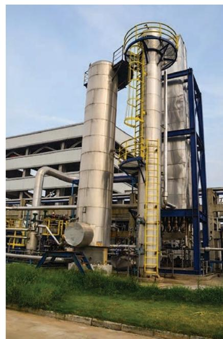
**FIG. 2.** The refinery’s WAR is used to reactivate spent powdered activated carbon from its PACT system.
