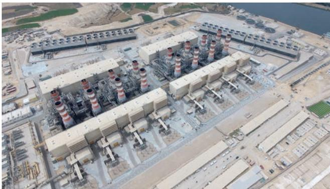
**FIG. 2.** Natural gas-fired CCPPs at Beni Suef in Egypt, each with a capacity of 4.8 GW.
