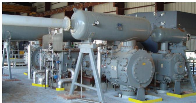
A typical Dresser-Rand HHE-VL reciprocating compressor installation utilizing an engine-type synchronous motor similar to the configuration of the three units that will be installed at a steam methane reformer in Texas.
