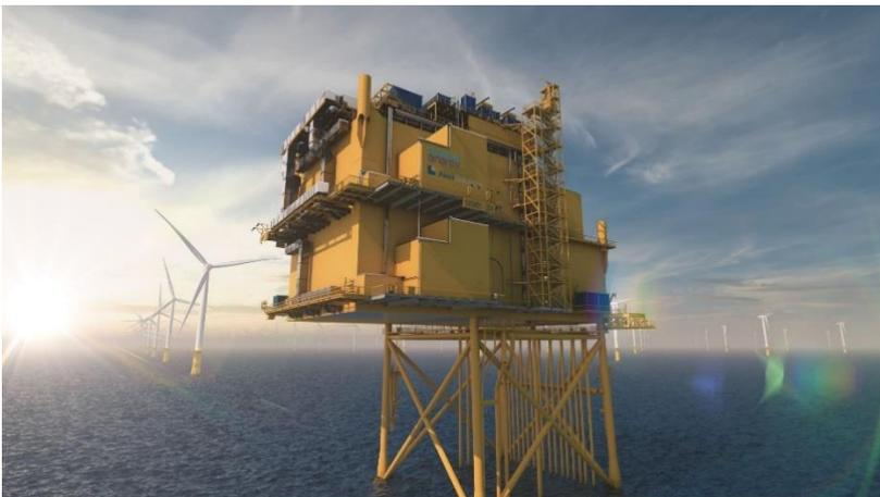
Picture description: The offshore converter station will collect the alternating current power generated by the wind turbines and transform it to direct current.
