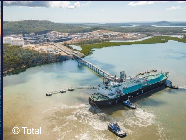
Siemens Energy will deliver equipment to its customer Total for the largest LNG project in Africa in Mozambique
