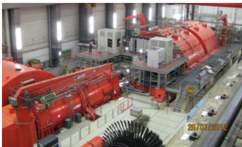
Bilibis - A Nuclear Power Plant converted to a Basic Rotating Grid Stabilizer
