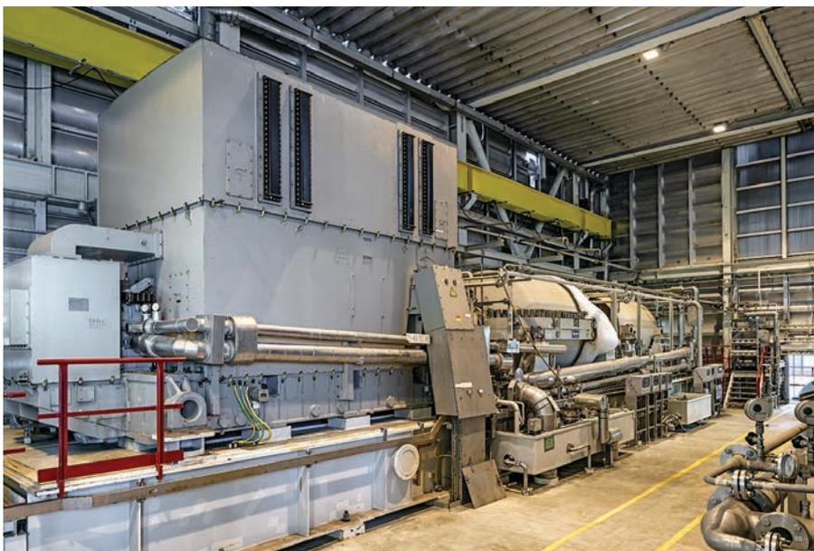
**FIG. 2.** The Hammerfest LNG terminal's three main refrigeration compressors are powered by all-electric drive trains.
