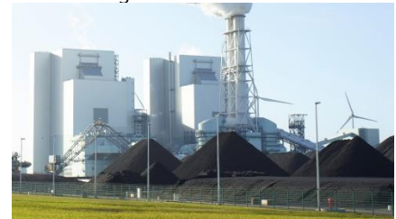
Eemshaven steam power plant.
