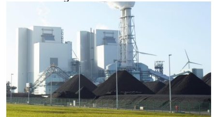
Eemshaven steam power plant.
