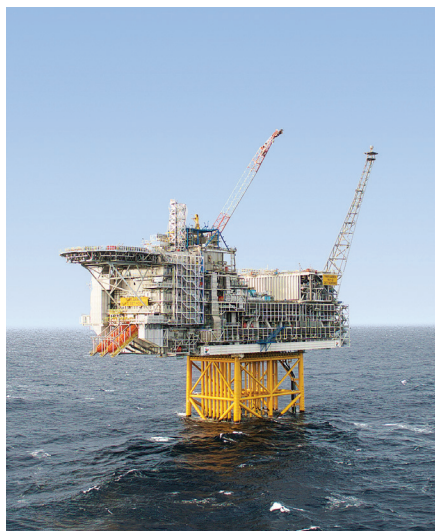
Fig. 1. Aker BP deployed remote CM on its offshore platform, built to develop Ivar Aasen field in the Norwegian North Sea, in an effort to reduce opex costs, increase regularity and improve operations safety.
