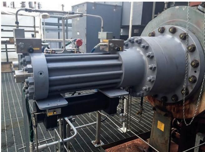
**FIG. 8.** An HVVCP unit installed on the outer end of a compressor cylinder used for hydrogen service.
