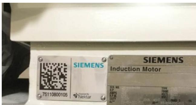
**Figure 1.** QR codes are used to access asset documentation from the field as well as maintenance and service histories.
