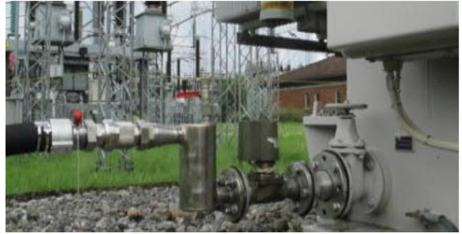
Installation for connection to the transformer tank bottom flange (from left to right): hose with dry disconnect coupling, air trap, solenoid valve, flange adapter DN80/DN40.
