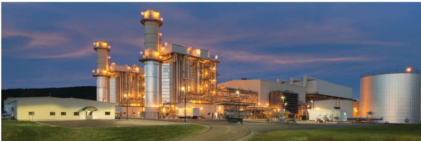
**2. Liberty for all.** The 829-MW Panda Liberty Power Project's single-shaft power plant blocks include two SGT6-8000H gas turbines, two SST6-5000 steam turbines, two hydrogen-cooled SGen6-2000H generators, and two heat recovery steam generators, along with the control system SPPA-T3000. Courtesy: Siemens
